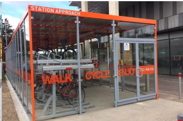
Figure 11: Station Approach Cycle Hub (Cyclepods, 2017)
